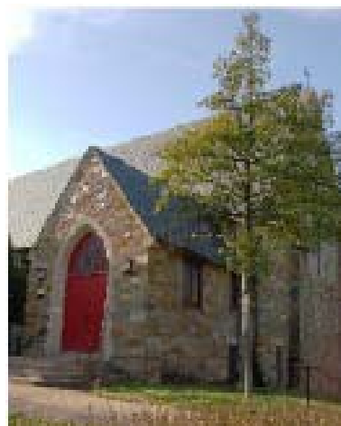
Front view of Wesley United Methodist Church, 5312 Connecticut Avenue (at the corner of Jennifer St, between Nebraska Ave. and Military Rd.)
